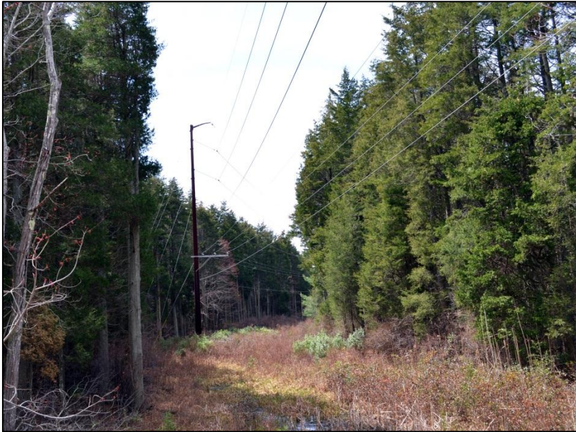
In 2004, the Commission entered into an agreement that permitted the construction of new power lines (as shown above) along a 33-mile corridor in the Pinelands Area.
